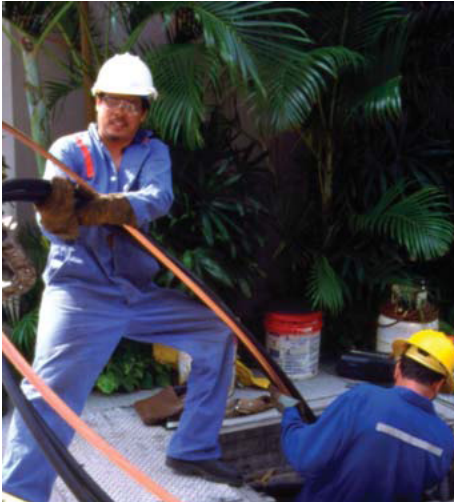
Hawaiian Electric underground crew replaces cables in downtown Honolulu.
