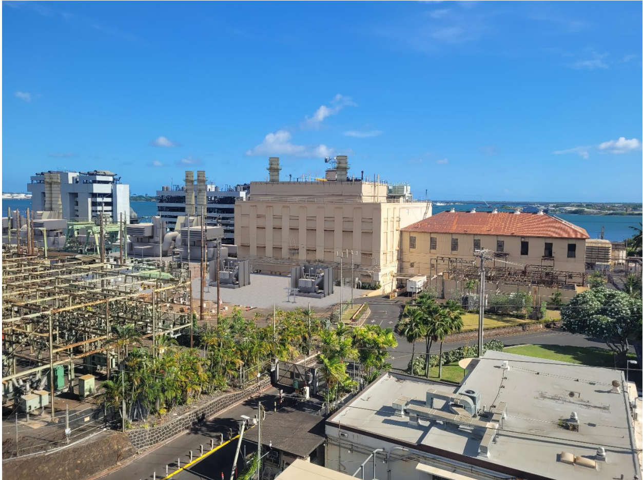
Above: Rendering of proposed Waiau Repower project, subject to change, when all six new units are in service. Image courtesy of Hawaiian Electric.
