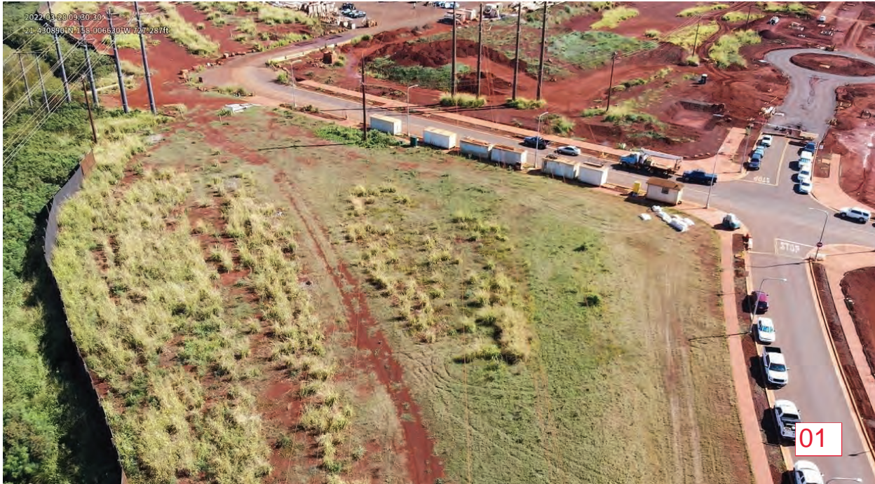
Existing 46kV overhead line
