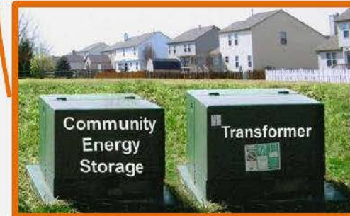
Distribution Grid Edge Storage 10's of kW (Li-Ion)
