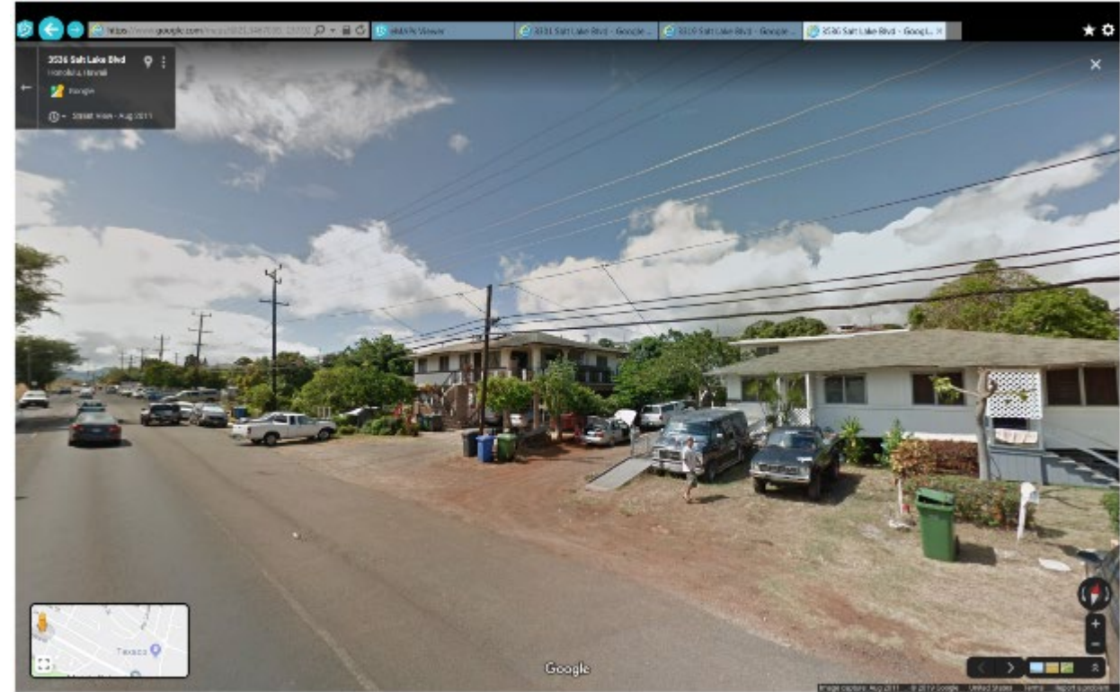
Loads are being served from OH lines along Salt Lake Blvd.
